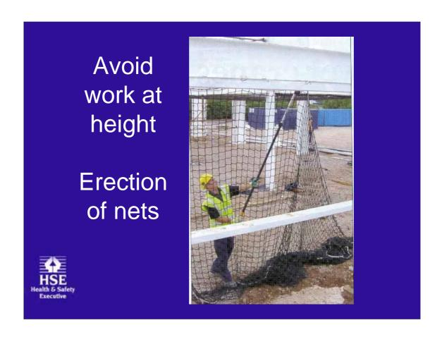
Installing nets from the ground using a rod and gripper system
