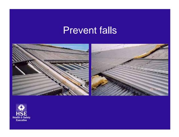
Coverings have been provided for fragile roof lights so that any foreseeable loading is being supported. Followed an accident when a person fell through an unprotected roof light.
