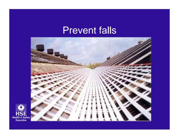
Protection either side of a valley frame gutter which can be used for occasional access
