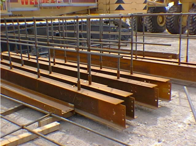
Steel beams designed with prefixed sockets to insert the edge protection at ground level and so preventing scaffolders being exposed to a risk from height
